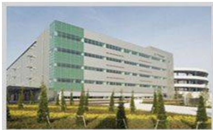
231–2 Nishimukojimacho Amagasaki–shi, Hyogo GLP Amagasaki 5Floor Floor Area: 11,774m 2
