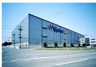
Logistics Center-East Japan
