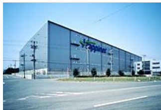
Logistics Center-East Japan
